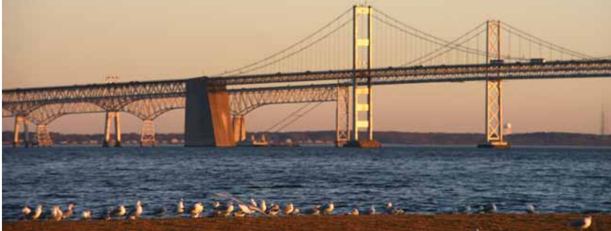
A view of the Chesapeake Bay Bridge from Sandy Point Beach State Park, Maryland.
