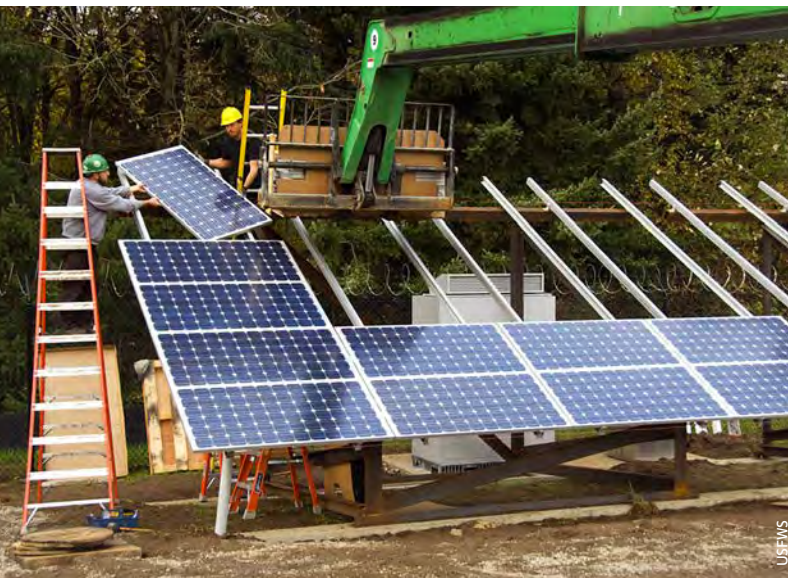
Solar panels under construction.
