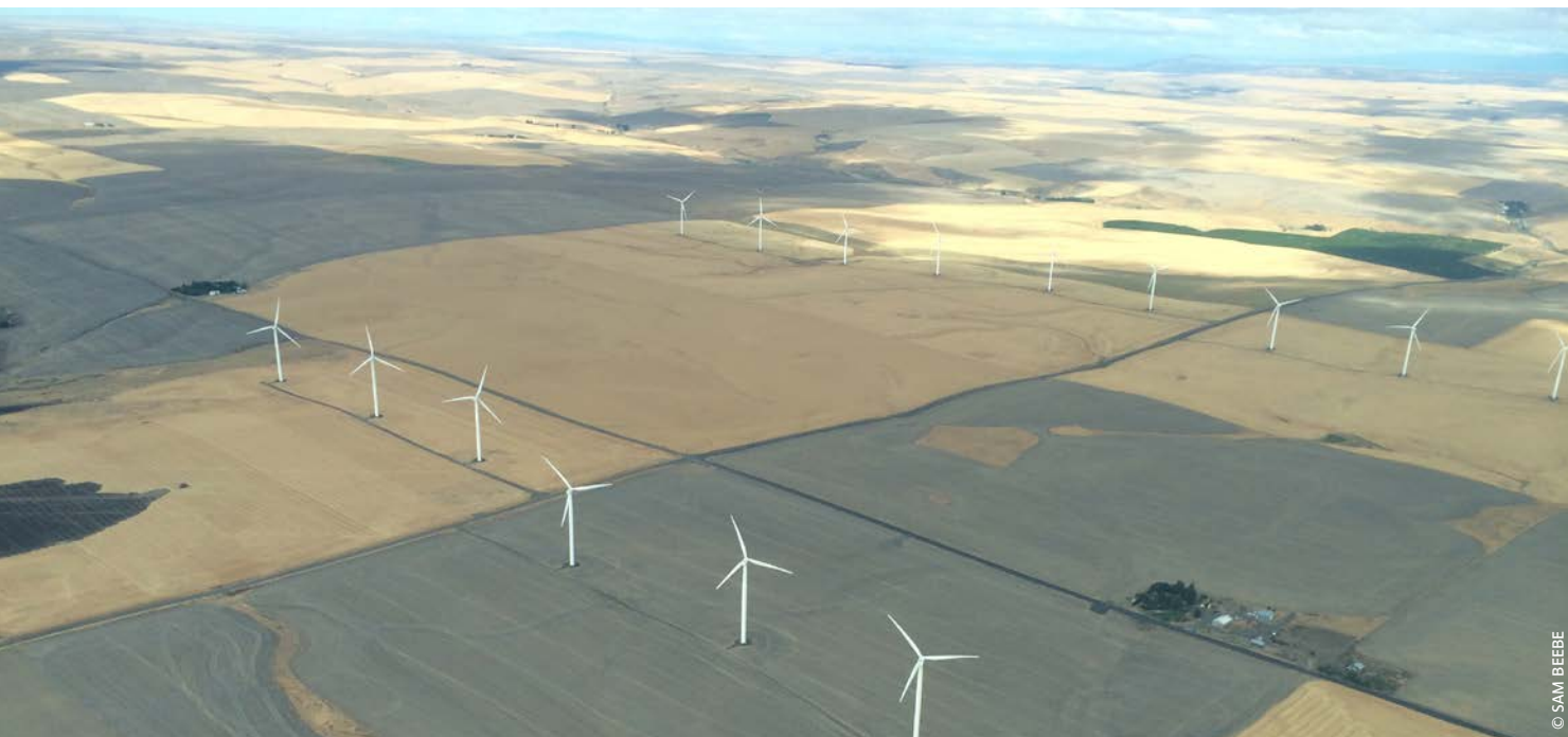
Aerial view of wind turbines in Oregon.
