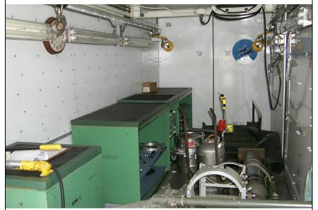
The interior of a WMT used at Kleine Brogel Air Base. Note the grey brace in the foreground used to lock in the bomb during maintenance. A logo for the Jabo G-34 fighter-bomber squadron at Memmingen Air Base in Germany is also visible on the inside of the right-hand side rear door.
