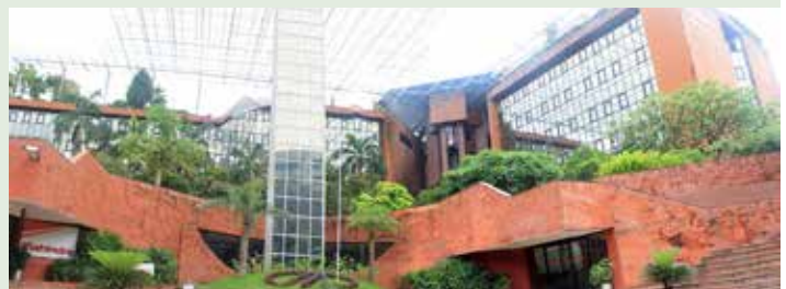
MAHINDRA TOWERS POST-RETROFIT.
