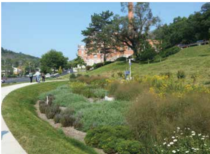
Bioinfiltration basin, Cincinnati Ohio.
