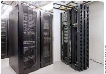
MDF room on floor 7 with traditional Cat 6 cable system (left) and IDF room on floor 8 with passive optical network (PON) system (right). Note that the fiber optic cables of the PON system dramatically reduce the amount of cable required as compared to the more traditional Cat 6 cable system.
