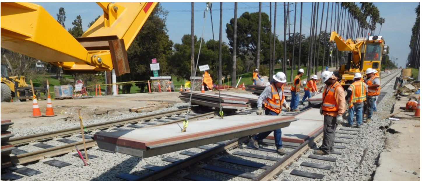
Installation of intersection crossing panels on the Crenshaw/LAX line.
