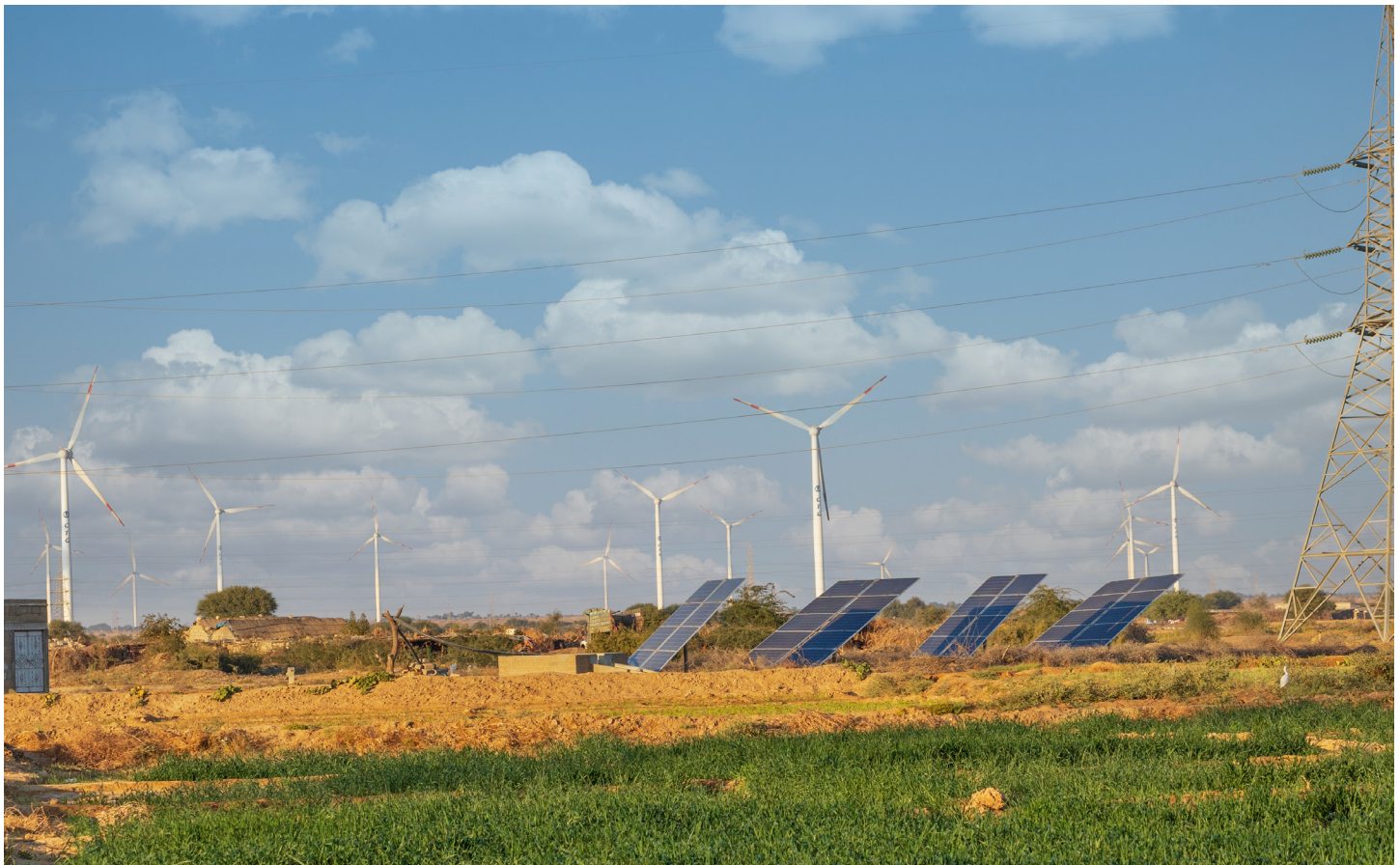
Wind turbines and solar panels in Jhampir, in Thatta District, Sindh, Pakistan.
