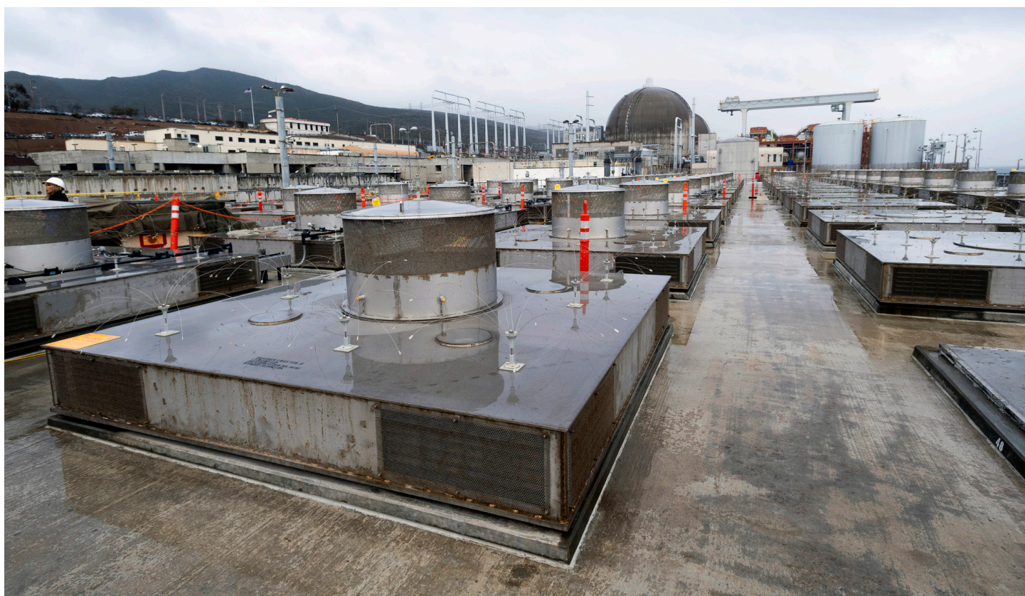
A Holtec HI-STORM UMAX dry storage system at the shuttered San Onofre Nuclear Generating Station.
