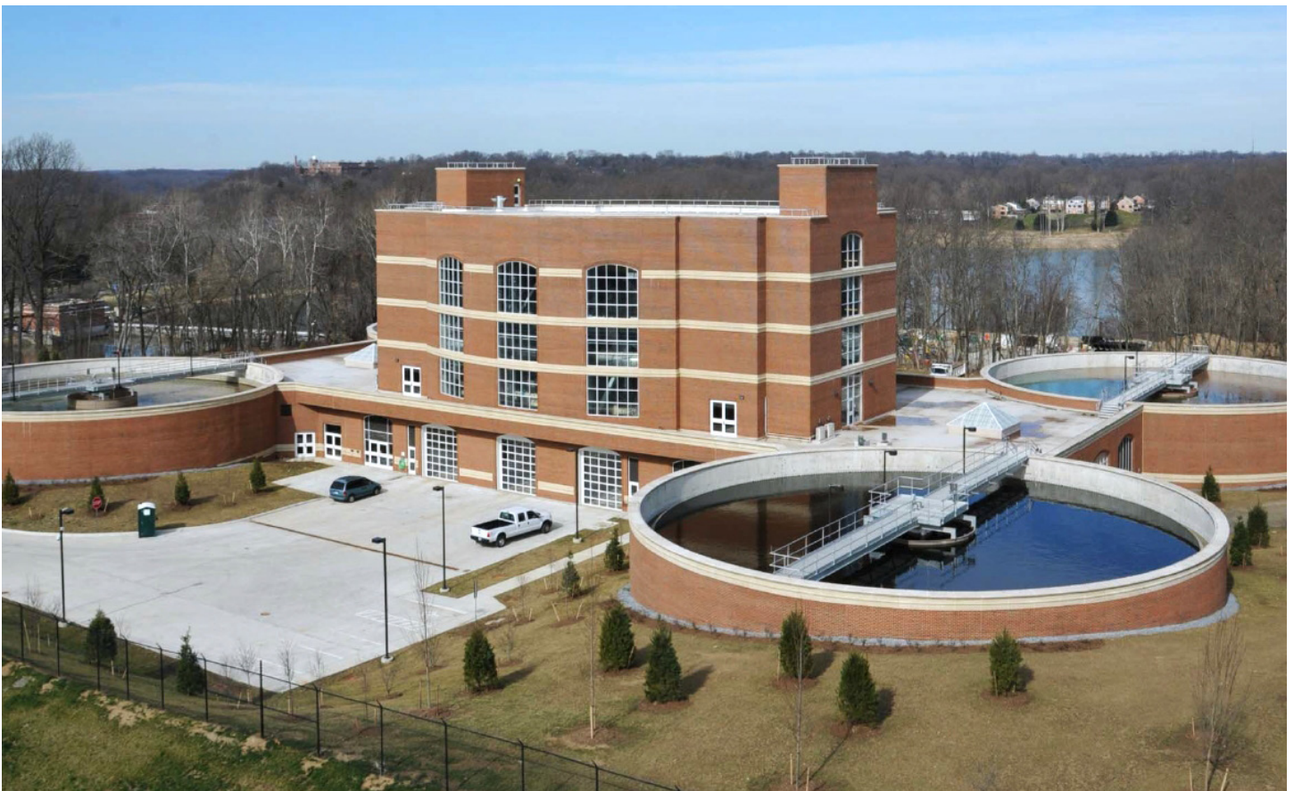
Drinking water treatment plant at the Dalecarlia Reservoir in Washington, DC.
