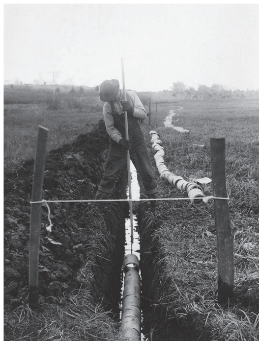
A History of Land Management Clay drain tile pipes were once laid by hand as shown in this historic photo (left) of early Minnesota farming. (Ayer, Harry Darius, circa 1910, Minnesota Historical Society) Modern equipment (right) like excavators and tile plows allows farmers to install perforated plastic piping quicker and easier.
