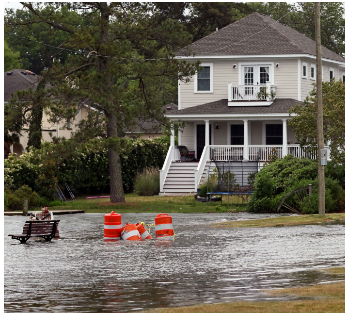
A road begins to flood as high tide moves into a residential neighborhood in Norfolk, Virginia, following days of rainfall.
