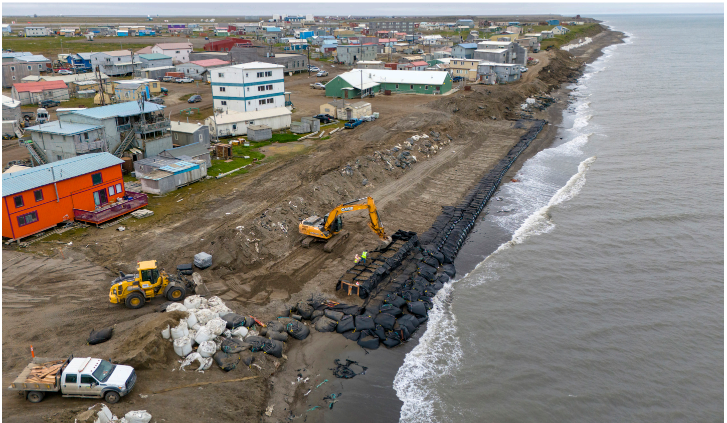
Reinforcement work being conducted on the sea wall in Utqiagvik, Alaska.
