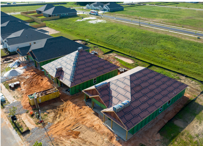
FORTIFIED Roofs™ being installed on newly constructed homes.
