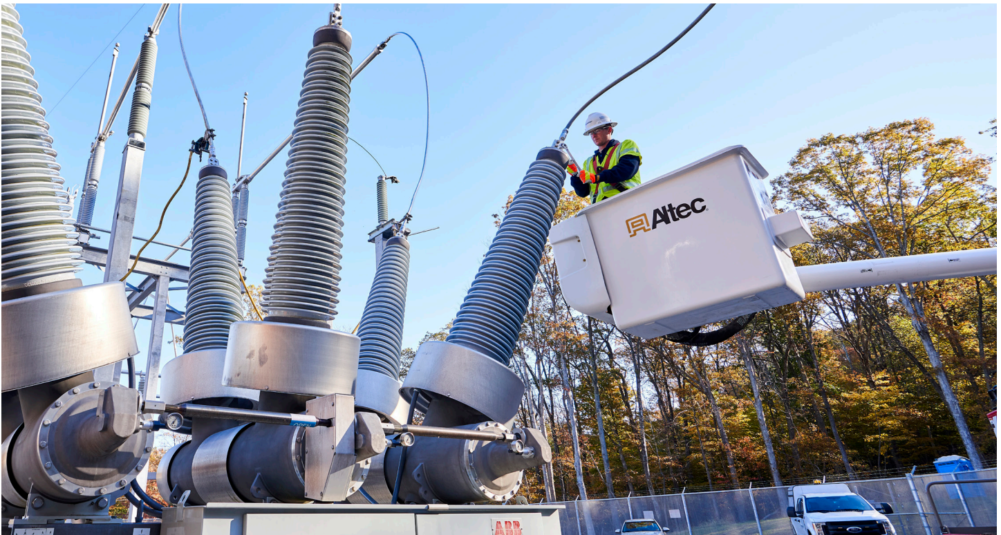
A Potomac Edison line mechanic working on a cable at a new electrical substation in Frederick County, Maryland, on October 24, 2019.
