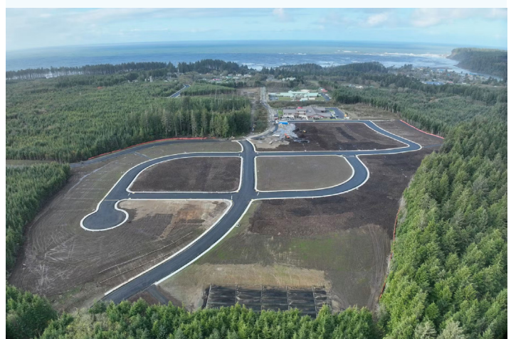
New streets, away from rising seas and tsunamis, await housing construction in the Quinault Reservation village of Taholah in November 2023.
