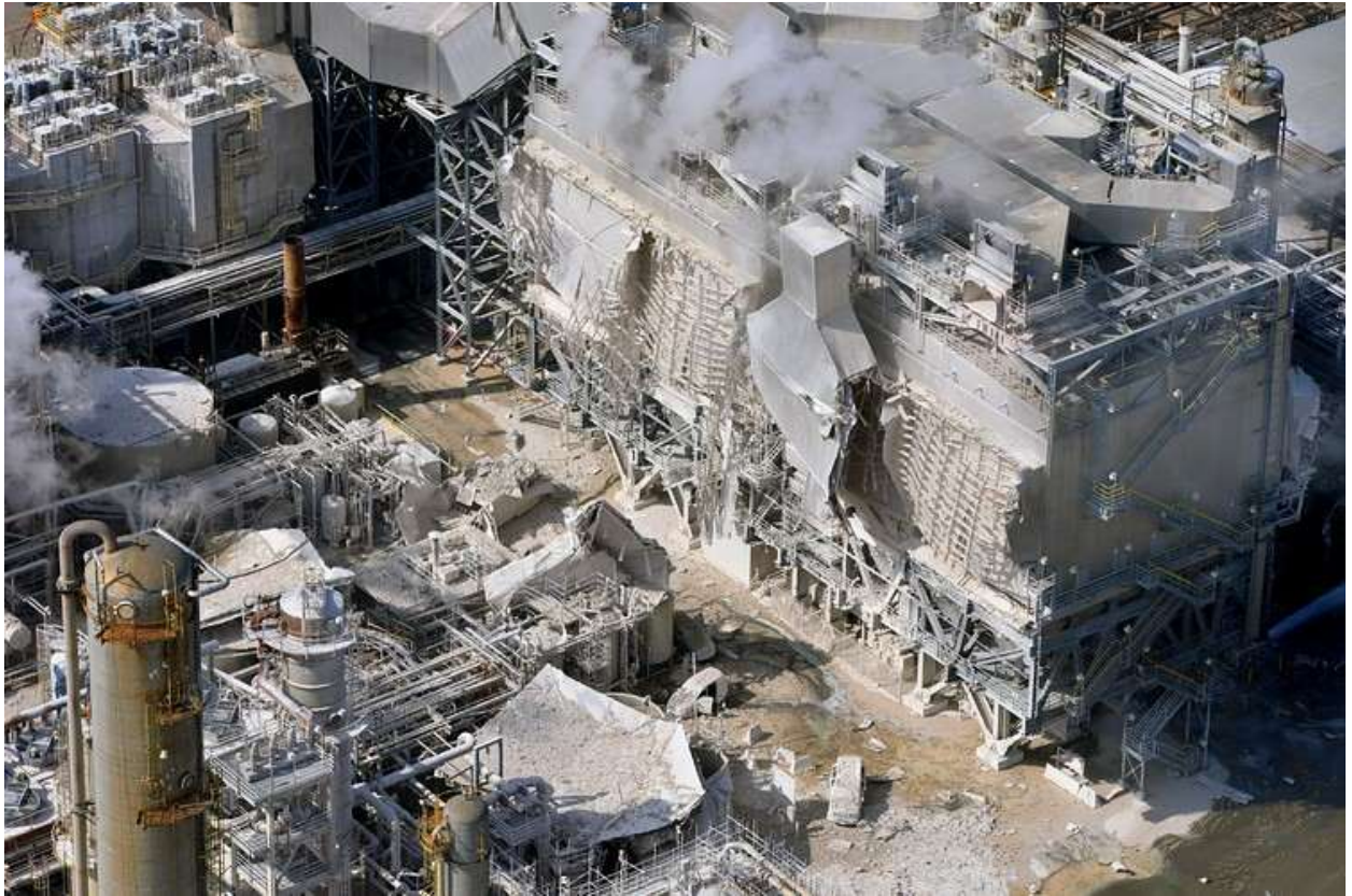
Torrance refinery after the ESP unit exploded, with damaged vehicle in the foreground. Photo: Associated Press (reproduced in Wall Street Journal, Explosion at Exxon Mobil Refinery Raises Gas-Price Fears , Feb. 18, 2015).
