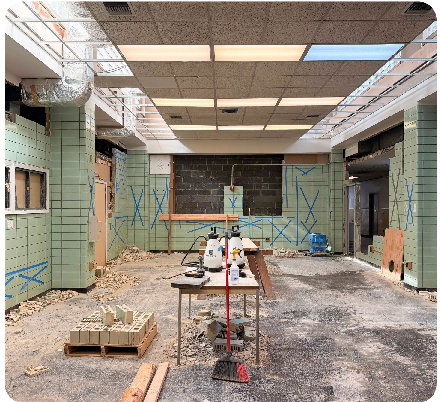
NYC School Construction Authority, source: CO Adaptive
