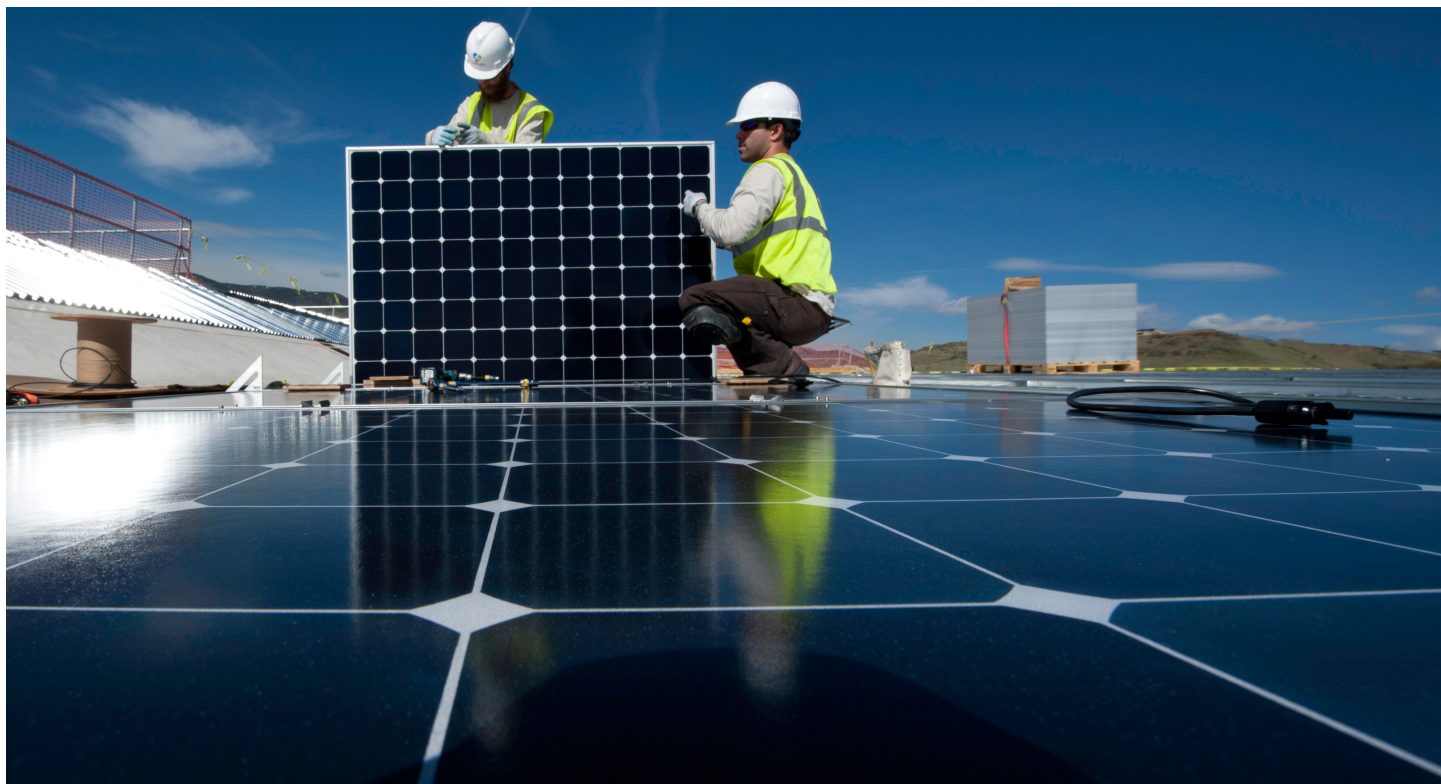
Workers installing one of 3,632 solar panel modules on the rooftop of the parking structure and south facade of the National Laboratory of the Rockies (NLR) in Golden, Colorado.
