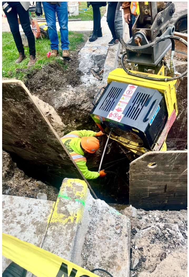
Lead service line replacement work in the Calumet Heights neighborhood on Chicago's South Side.
