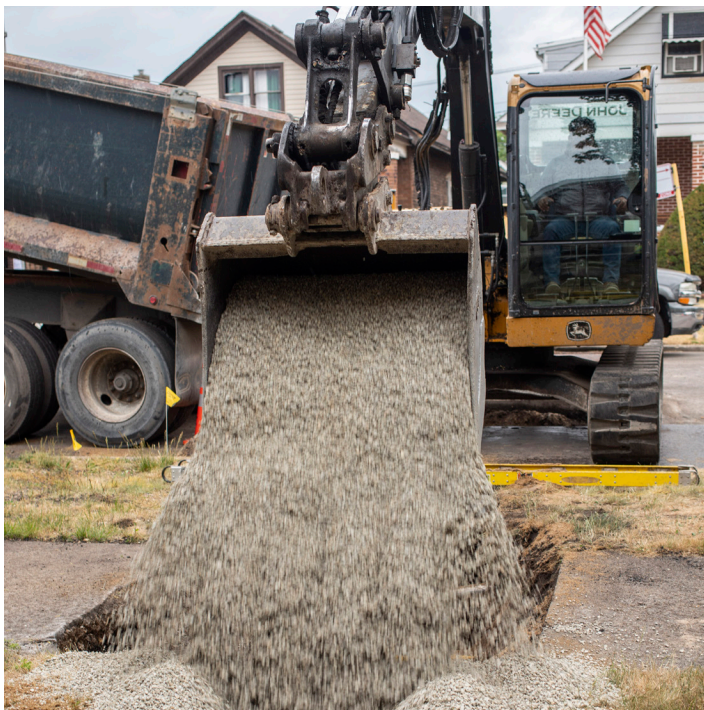
A construction worker using an excavator to fill in a ditch after replacing a lead service line.
