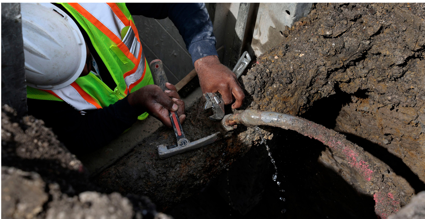
A contractor fixing and closing off a leaking lead service pipe ahead of replacement work on Chicago's West Side.
