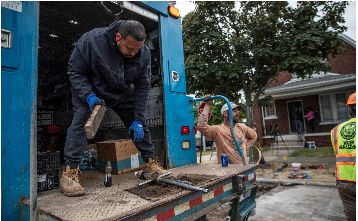
A construction worker gathers tools during lead service line replacement work in the West Roseland neighborhood of Chicago.
