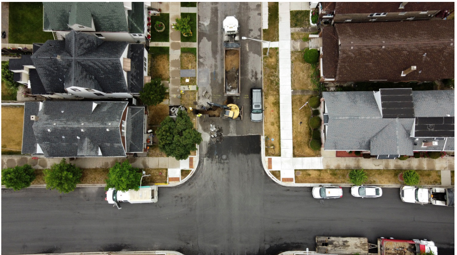
A construction crew using an excavator during replacement of a lead service line in the West Roseland neighborhood of Chicago.
