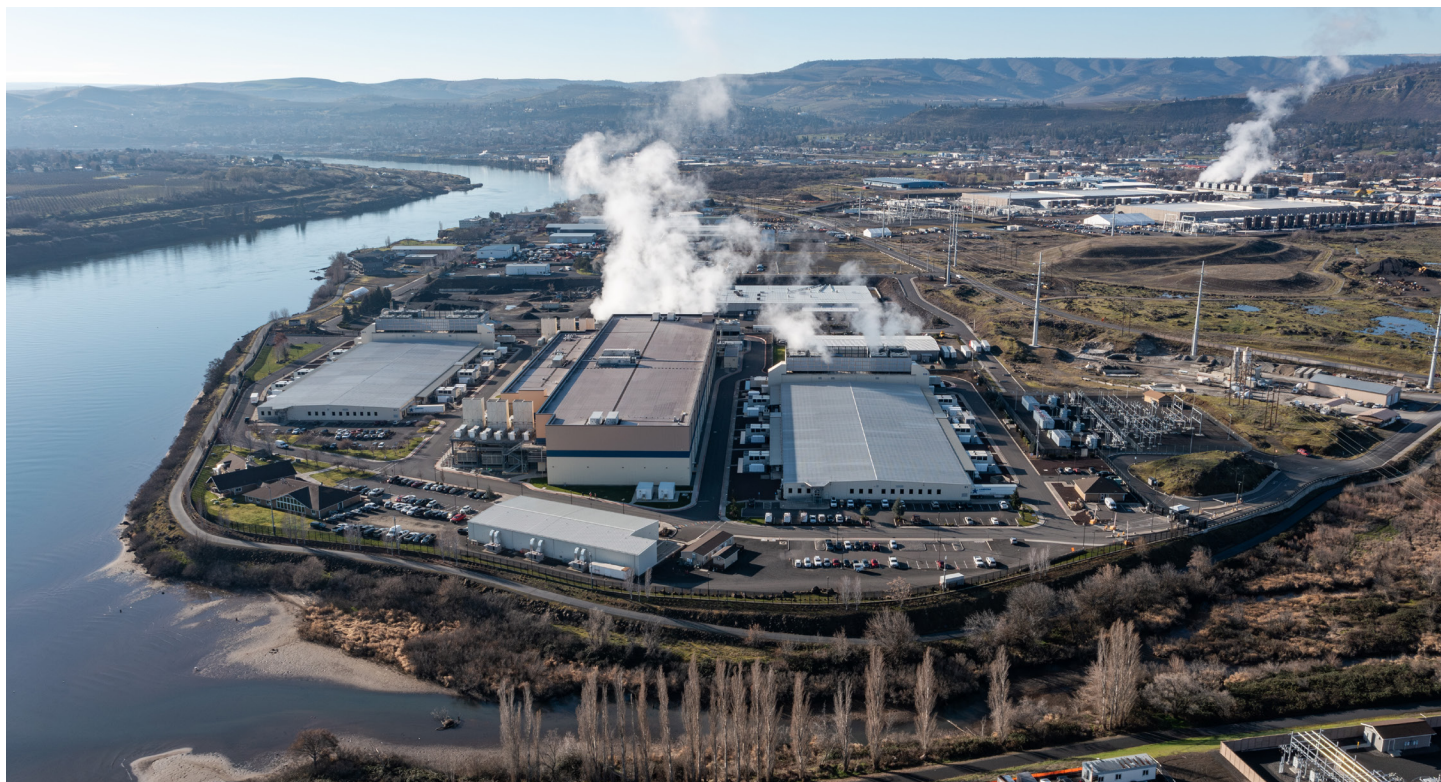
A massive hyperscale data center campus, located along the Columbia River in The Dalles, Oregon, USA.
