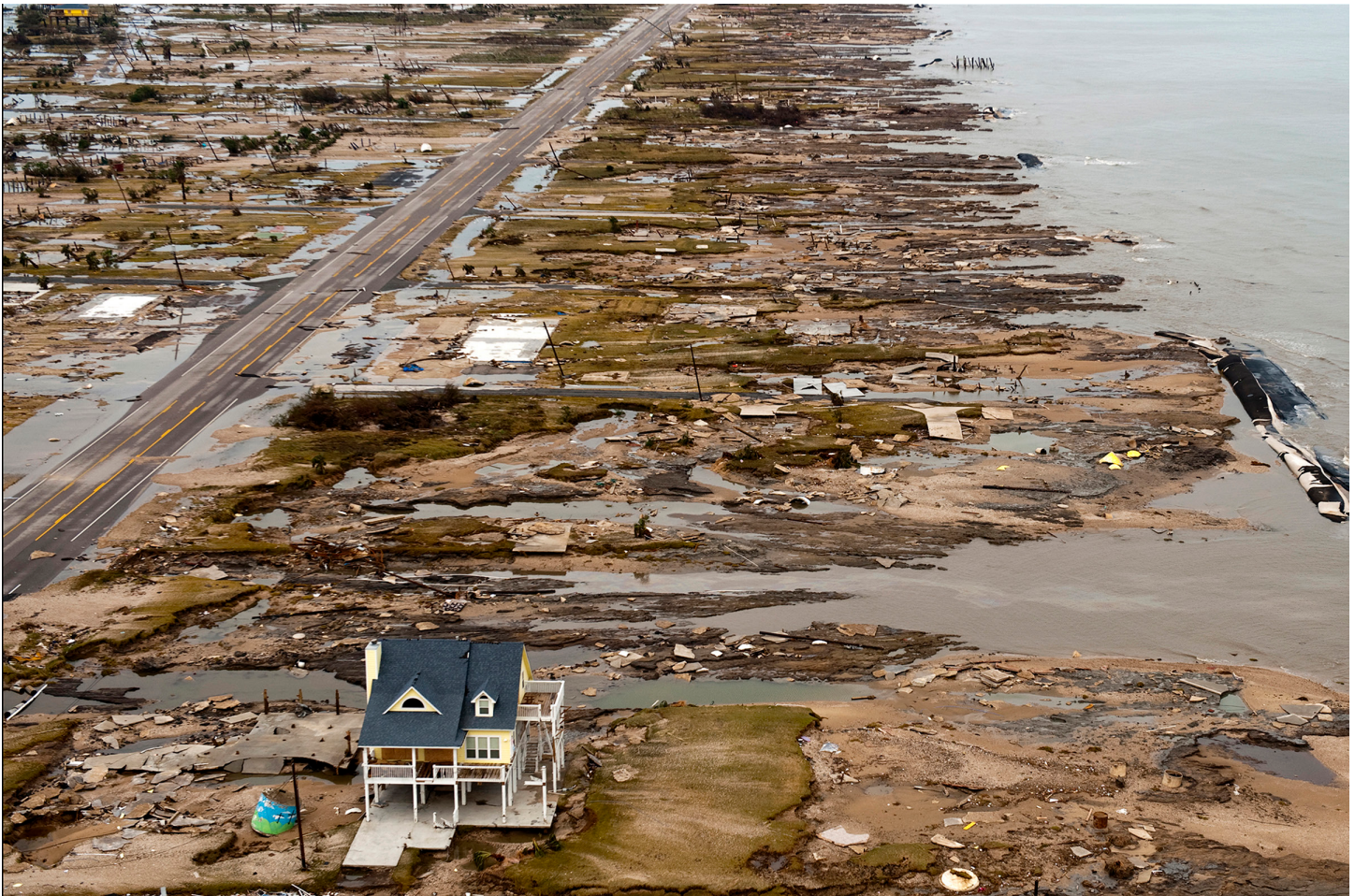
NCIUA's FORTIFIED program was partially inspired by the survival of this home in Gilchrist, TX after Hurricane Ike in 2008. By implementing risk reduction measures at scale, state-created insurers can significantly reduce claims after major disasters.
