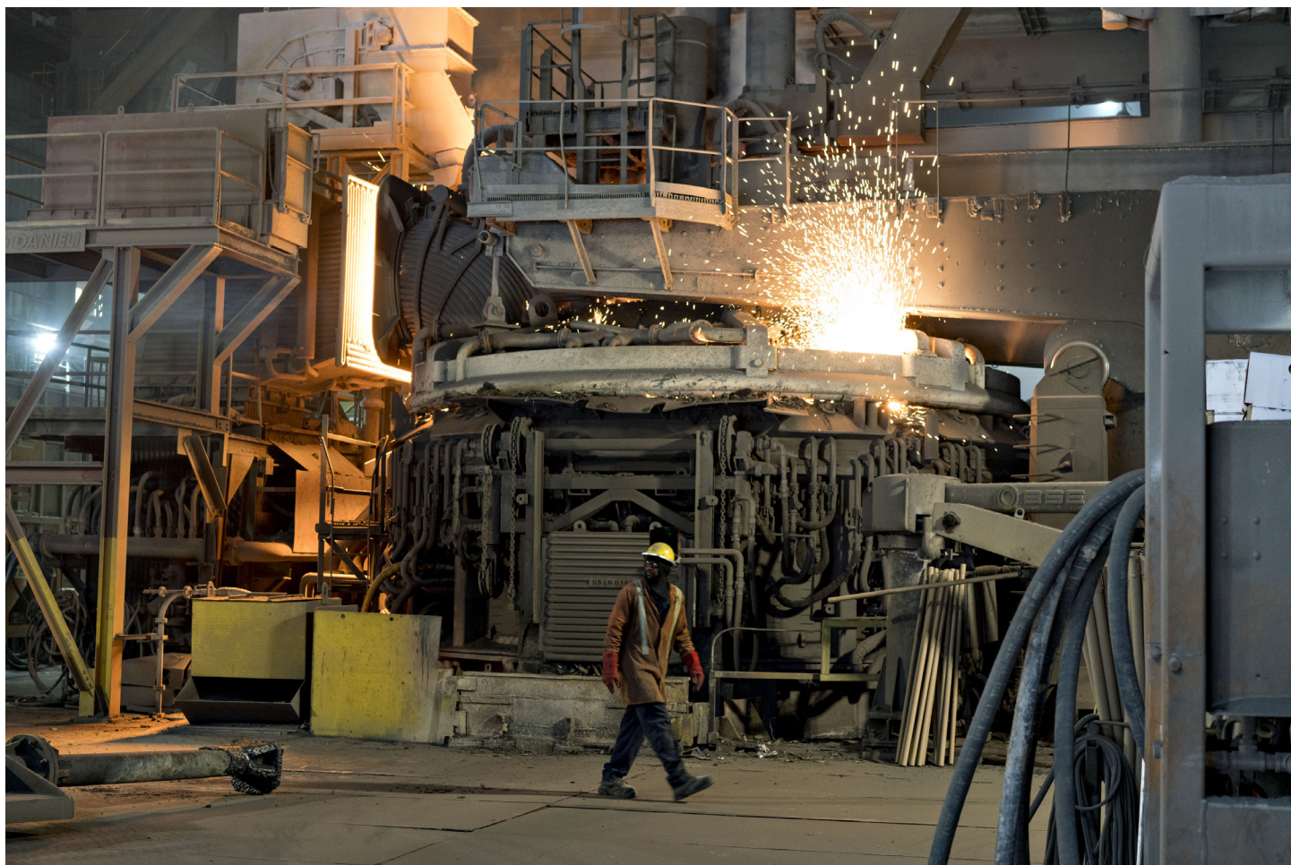
An electric arc furnace at the NLMK Indiana facility in Portage, Indiana.
