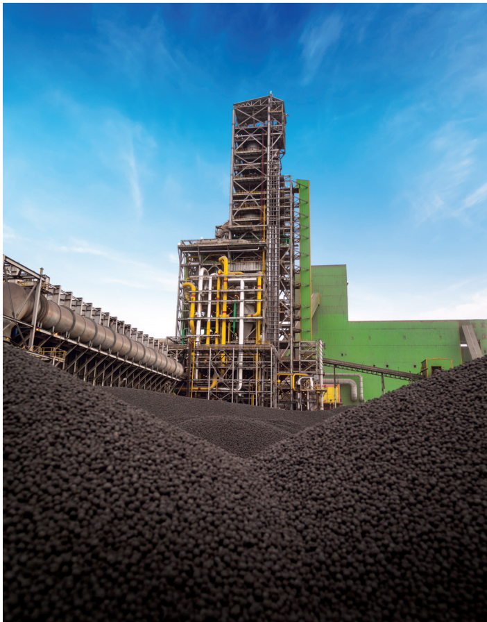
The MIDREX® Module 2 DRI shaft furnace at the Tosyali Algeria complex in Oran, Algeria. This plant is tied for the largest single module DRI plant in the world with a capacity of 2.5 Mtpy.
