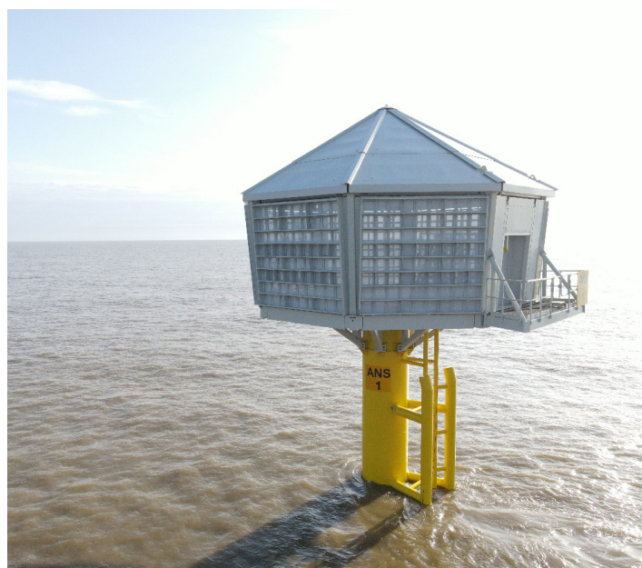
Three nearshore artificial nesting structures installed by Red7Marine along the East Coast of England on behalf of Ørsted. The structures are required as a part of the Development Consent Order for the Hornsea 3 Offshore Windfarm as an ecological compensation measure for a vulnerable seabird species—the Black-legged kittiwake ( Rissa tridactyla ).
