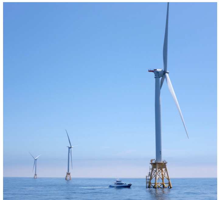
A vessel approaches the base of a turbine on Block Island Wind Farm, located in the Atlantic Ocean off the coast of Rhode Island.
