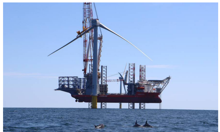
Dolphins swimming as a wind turbine installation vessel builds an offshore wind turbine on top of a previously installed foundation.
