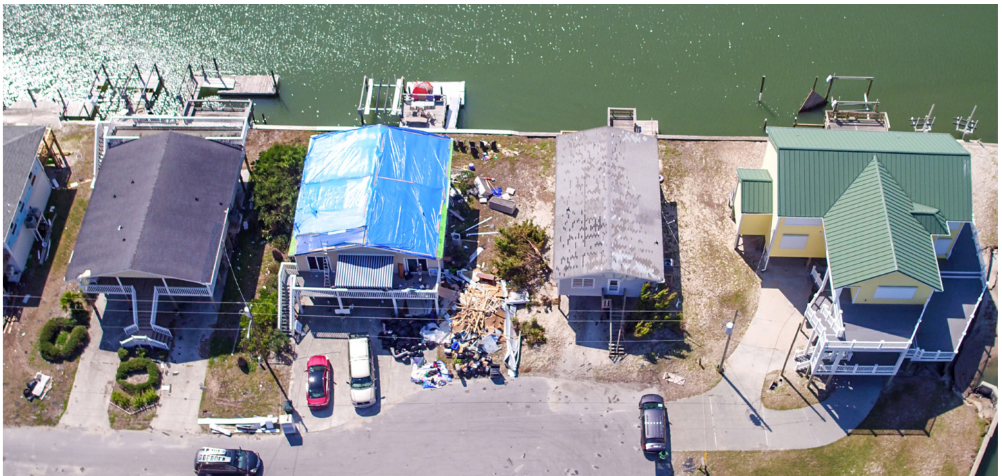
The yellow house on the far right with the green roof is FORTIFIED. NCIUA's investments in FORTIFIED roofs reduce the amount it pays out in claims after hurricanes and severe storms.
