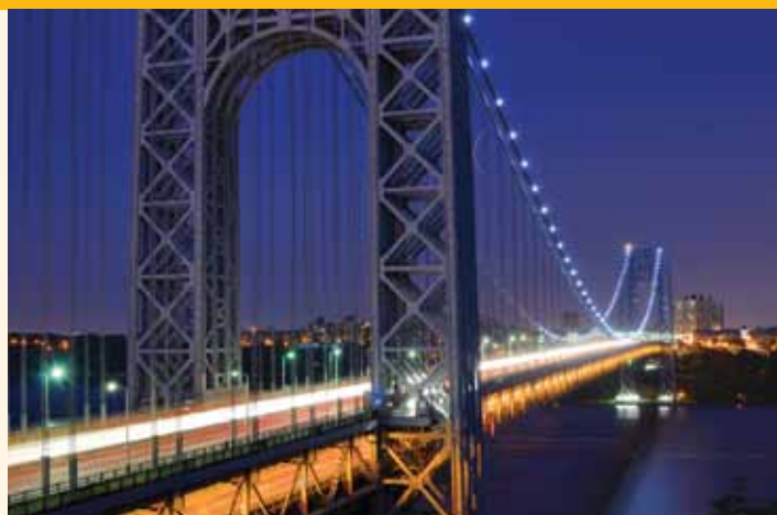
LSI Industries' LED lighting, featured here on New York's George Washington Bridge, creates good jobs in Ohio while saving money for municipalities and businesses.
