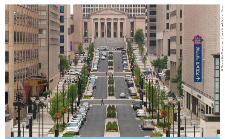
Nashville completed one of the first green streets in the Southeast, transforming a major downtown road into a pedestrian-friendly corridor by incorporating sidewalk-level bioretention planters, bioretention curb bump-outs, a landscaped median, porous concrete sidewalks, and planting 102 shade trees.
