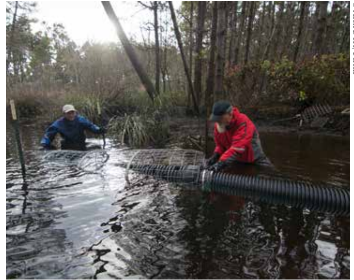
Positioning the intake assembly on a beaver deceiver, Oregon.
