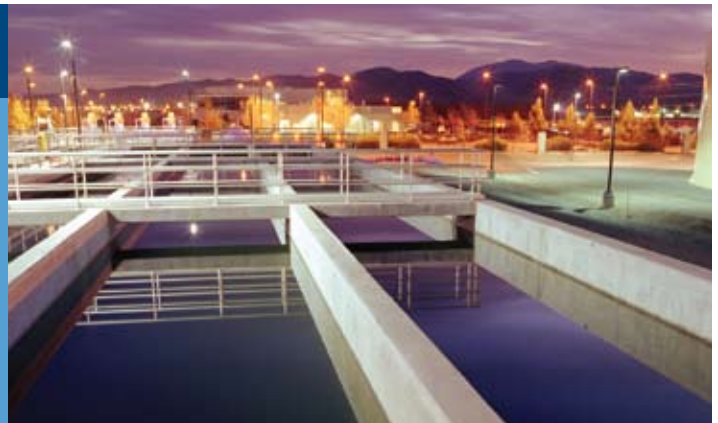
A water recycling facility at the Delta Diablo Sanitation District.
