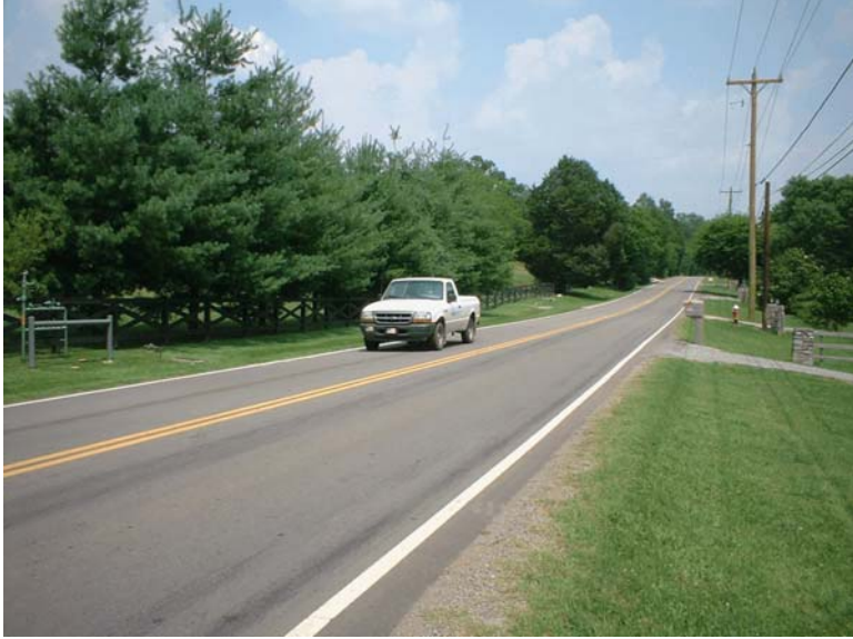
Typical collector street.
