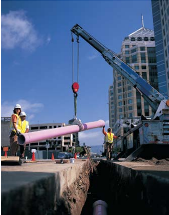
This "purple pipe" being installed by EBMUD will deliver recycled water to customers.
