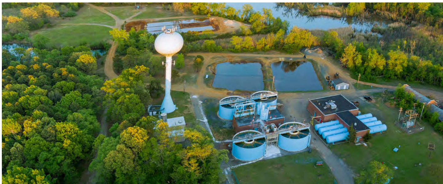
Aerial view of a wastewater treatment facility.
