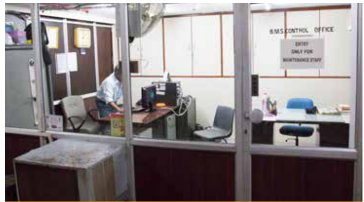
The building's management system control office
