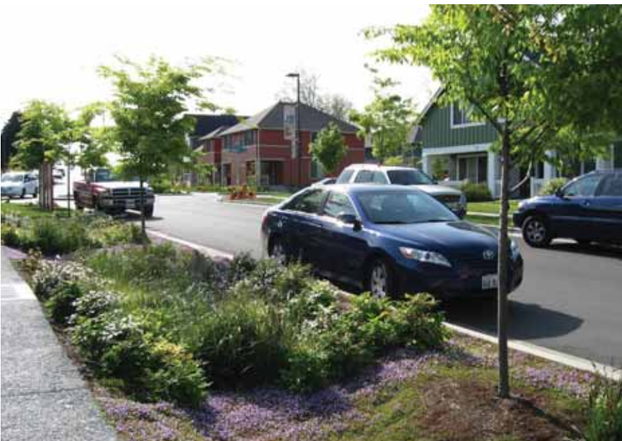
Drainage swale, shown here in Seattle, captures rainwater and reduces pollution
