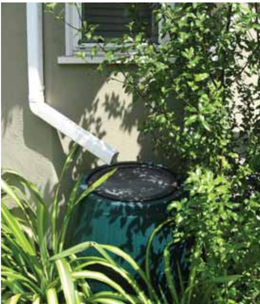
Rain barrels, such as this one in Santa Monica, California, capture rainwater for the garden
