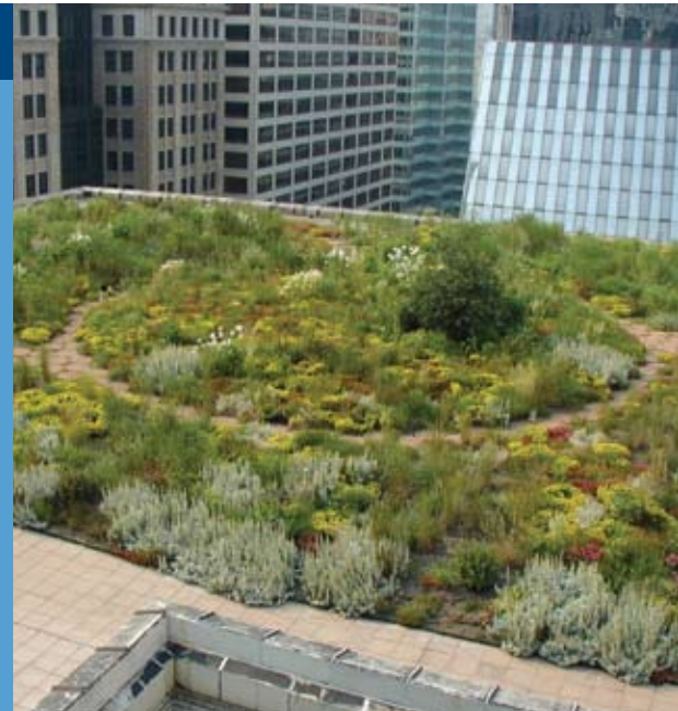
Photo courtesy of Roofscapes, Inc.
