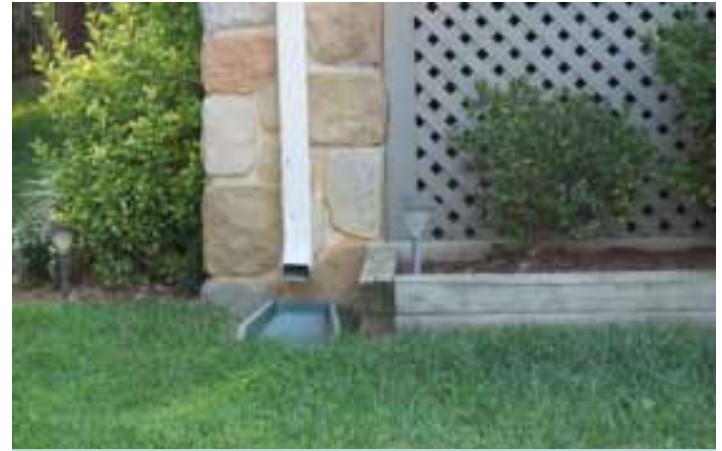
This downspout disconnection drains to a grassy area that absorbs the runoff into the ground.
