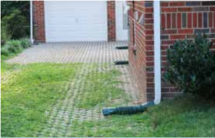
This downspout disconnection drains to a driveway with pervious pavement. Pervious pavement allows the rainwater to soak into the ground instead of running off.
