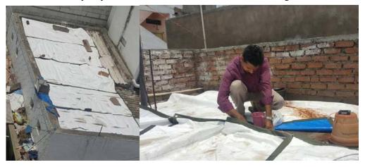
Figure 14: Pictures showing cool roof pilot installation and testing underway in Hyderabad, May 2017 (ASCI-IIIT)
