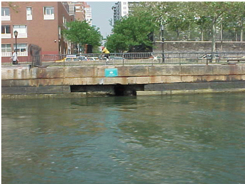
Photo 8: View of a CSO outfall.
