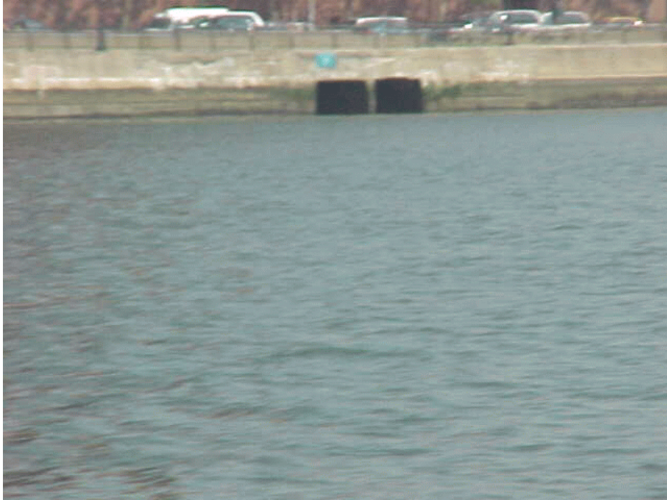
Photo 7: View of a CSO outfall.
