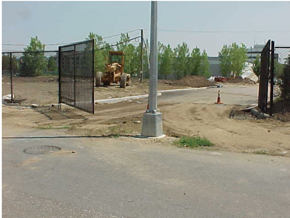
Photo 5: View south, from 15th Avenue, of entrance to the construction site.
