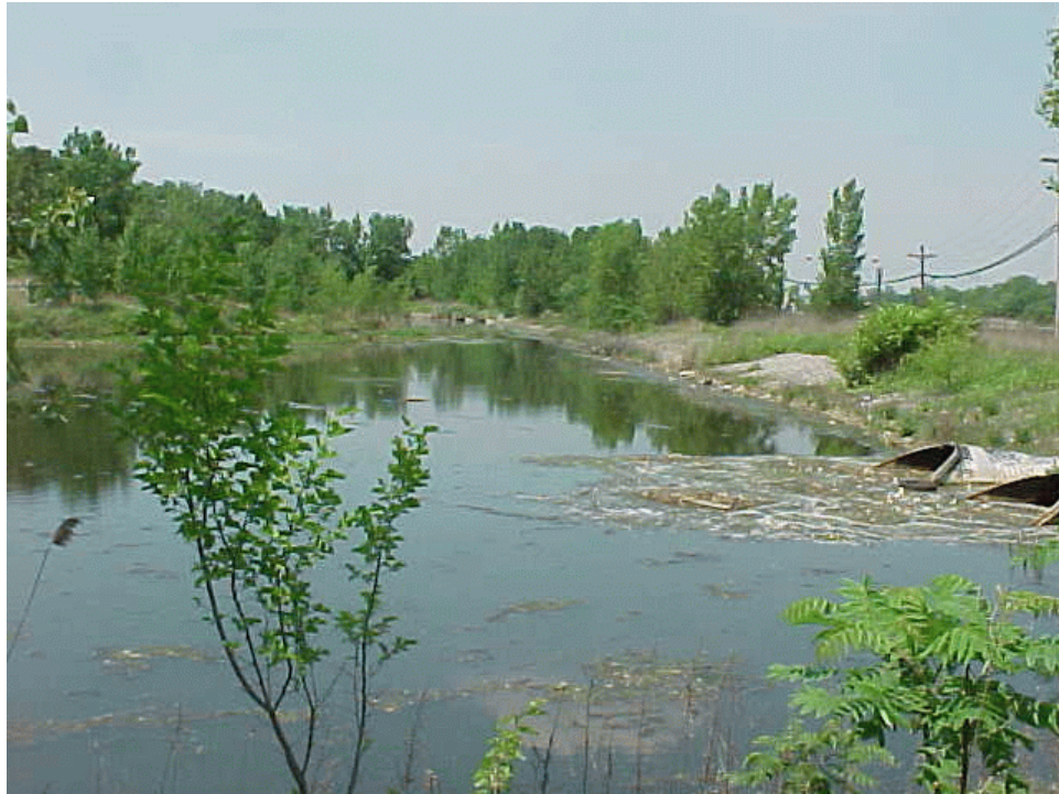
Photo 3: View north along the portion of the detention basin that parallels Linden Place.
