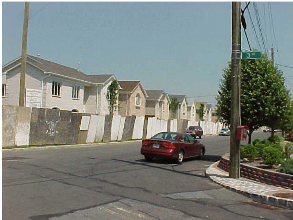
Photo 8: View east along Powell's Cove Boulevard.
