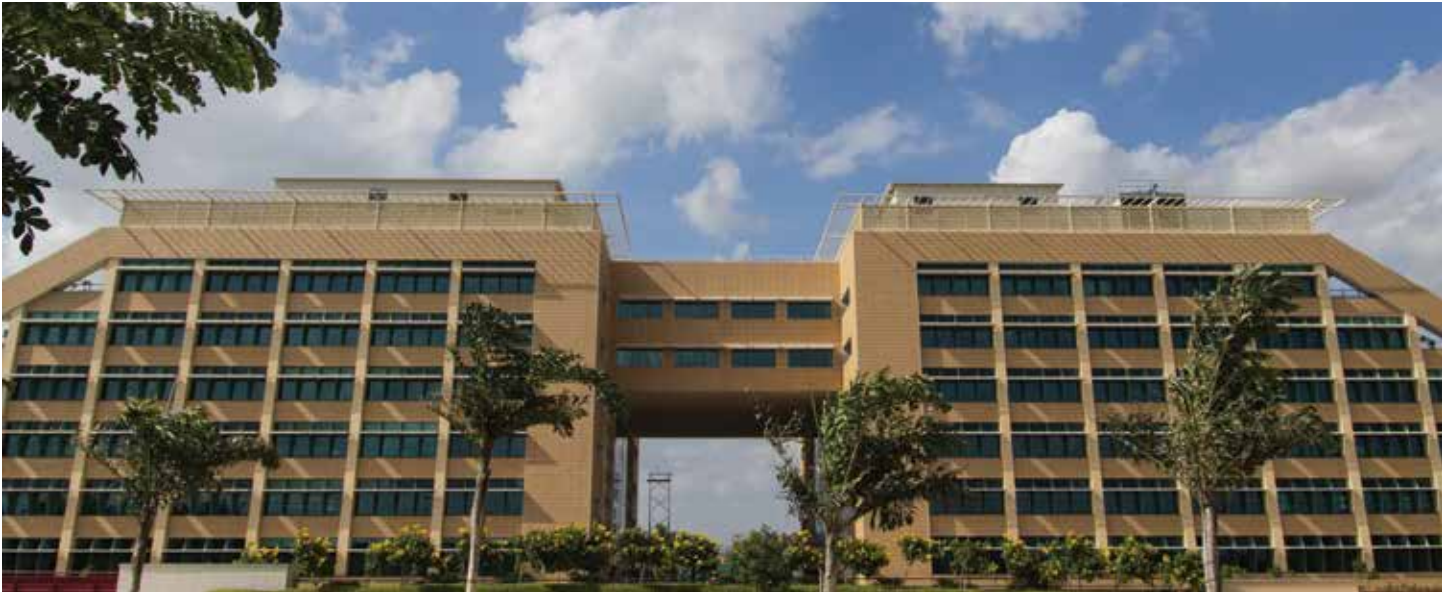
Exemplifying a market champion, India's first commercial radiant-cooled building, Infosys Software Development Building, located in Hyderabad, Andhra Pradesh, India.
