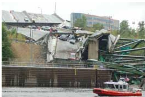
Delayed maintenance led to the collapse of the I-35W bridge, north of Minneapolis, in 2007. Kevin Rofidal, United States Coast Guard
