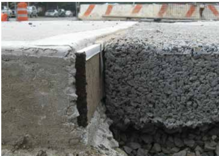
Porous concrete sidewalk Paerdegat Basin, CSO Detention Facility, Brooklyn, New York.
