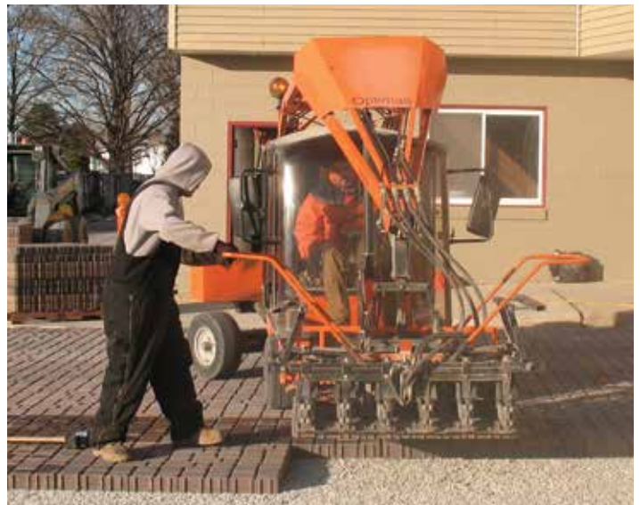
Installation of porous pavers at the Energy Exchange (November 2009).
