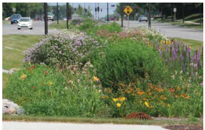
Bio-retention swales for stormwater treatment along Grange Avenue in the Village of Greendale, Milwaukee.
